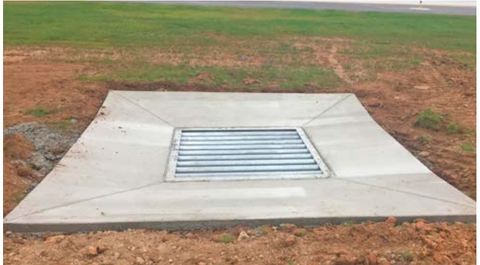
Airport steel galvanized pipe grates for taxiway drainage.
