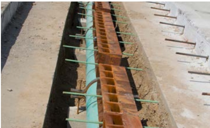
Linear slotted drain vane grate during installation
