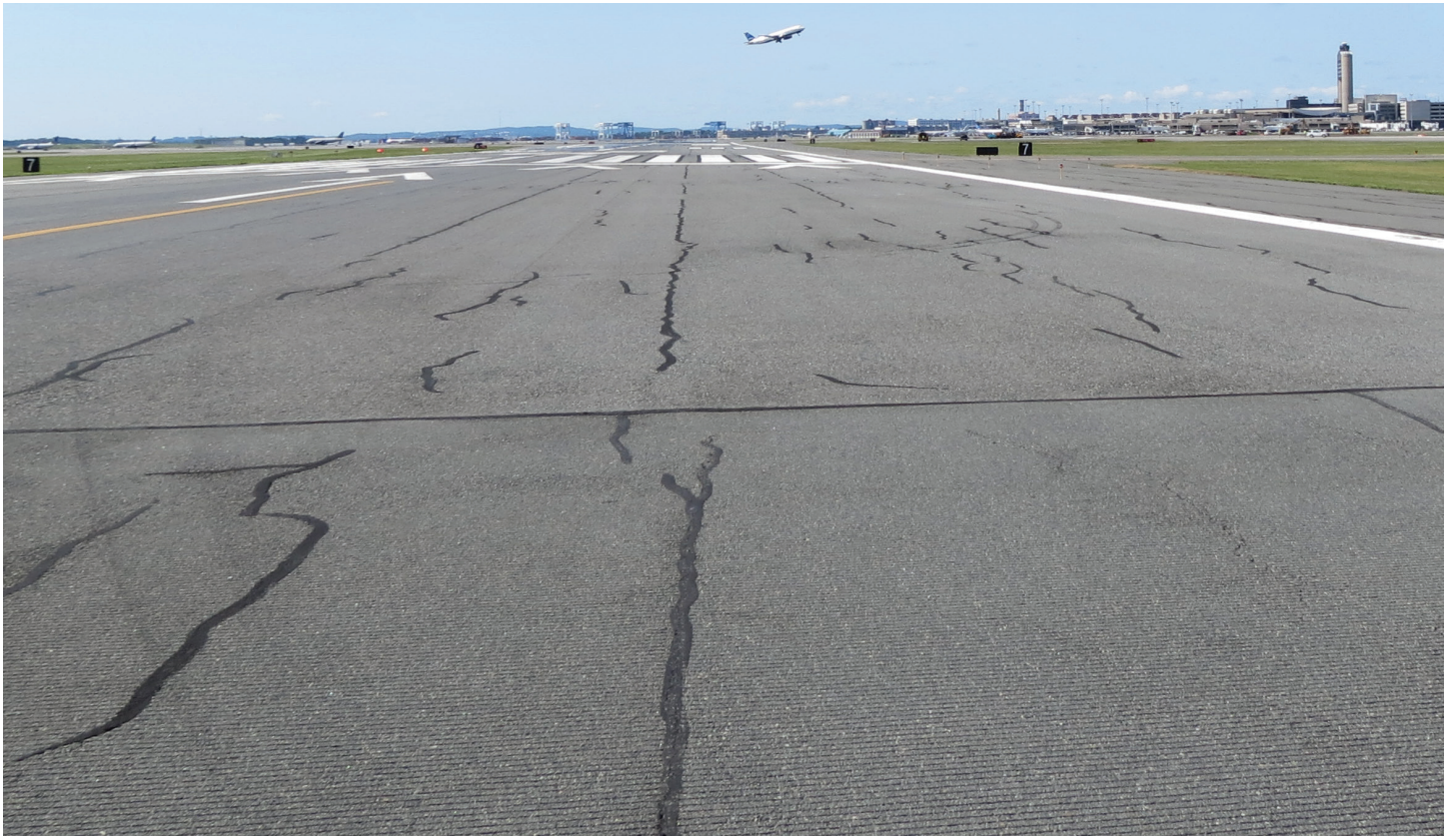
Logan International runway ten years after being repaved with a P-401 mix (above) and a P-404 mix with StellarFlex FR ® (below). Both were installed at the same time.
