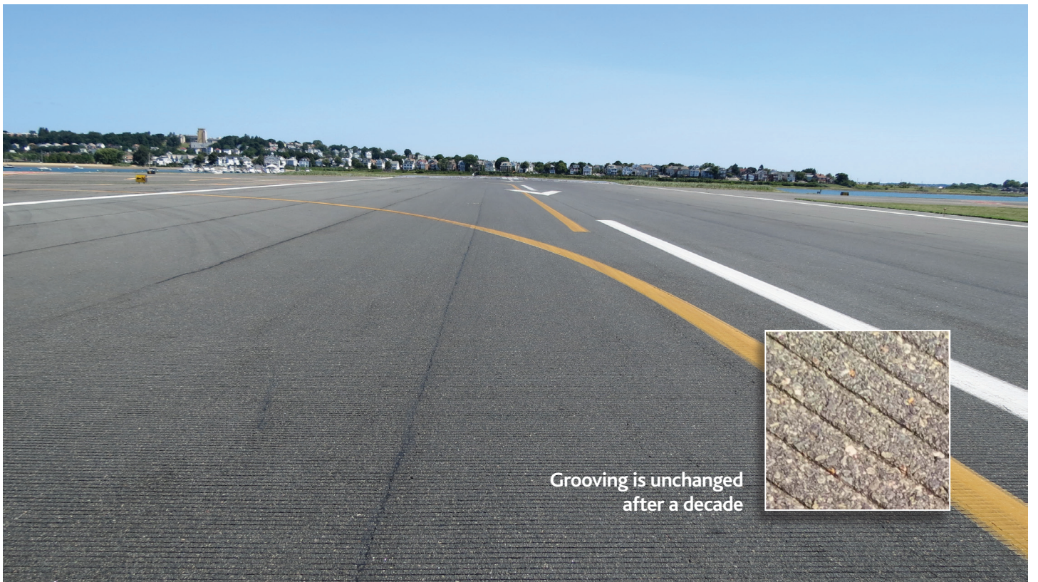
Logan International runway ten years after being repaved with a P-401 mix (above) and a P-404 mix with StellarFlex FR ® (below). Both were installed at the same time.
