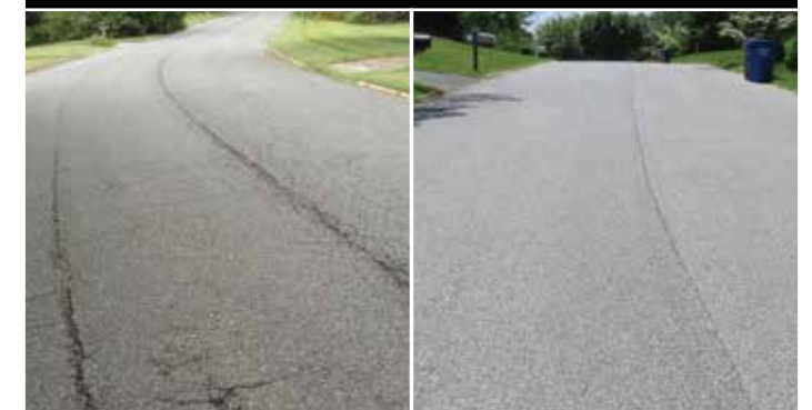
Kreitler Road in Harford County, MD, before (left) and 9 years after (right) installation of FlexGard®
